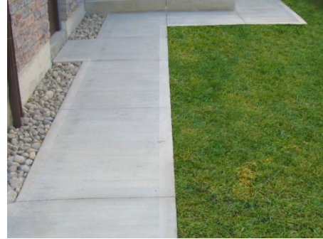
Brushed Concrete Footpaths
